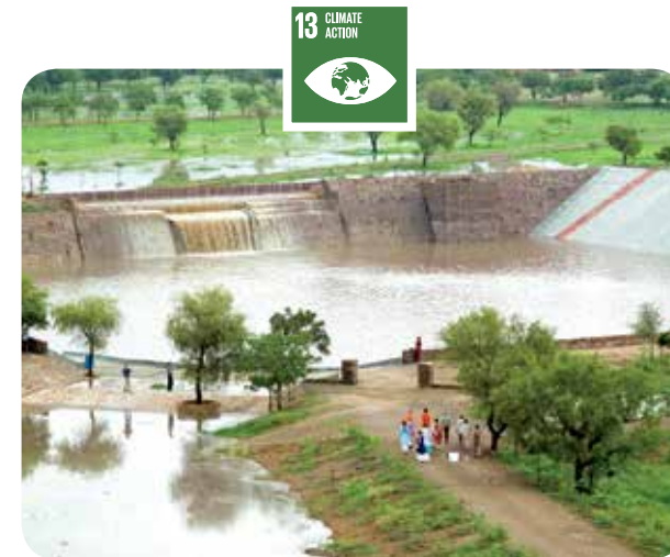
Desert Rainwater Harvesting Project
