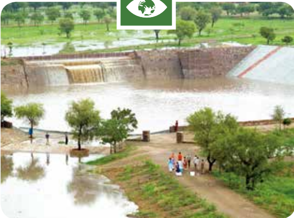
Desert Rainwater Harvesting Project
